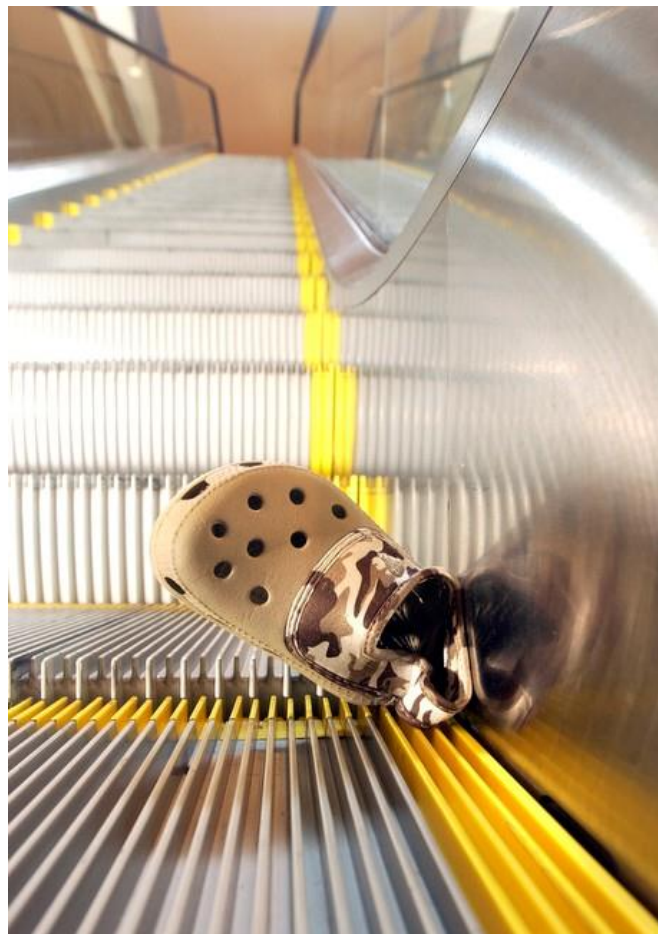
Figure 4 Side-of-step entrapment with raised step edge profile
