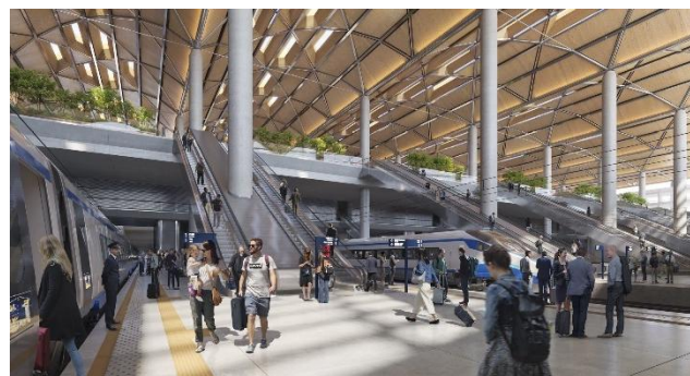
Figure 3 – N+1 Redundancy design and 3 flat steps escalator at CPK airport hub
