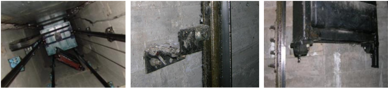
Figure 3 Lift damage of the Van Earthquake [6]
