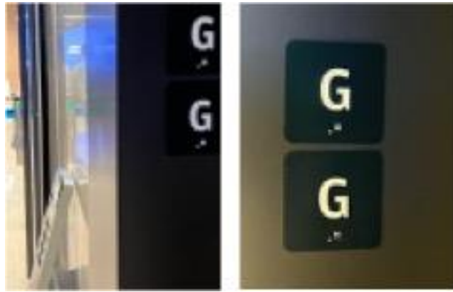
Figure 3 Confusing Nomenclature Signage – one G pertains to the floor number while the other pertains to the lift identification
