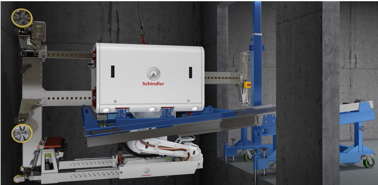
Figure 5 Safe moving of Schindler R.I.S.E into hoistway
