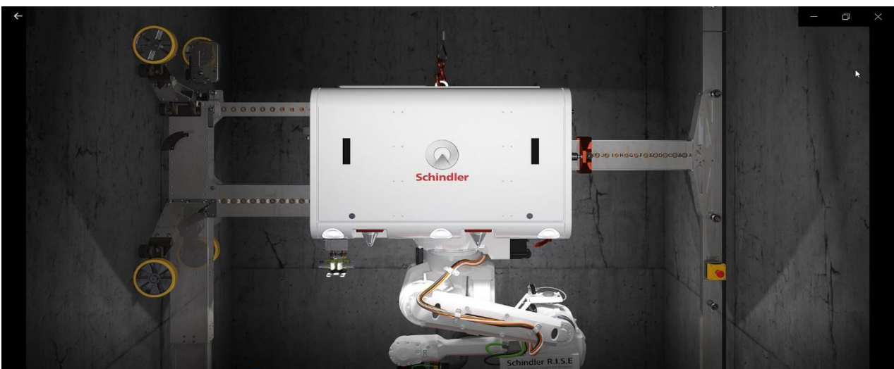
Figure 6 Automatic vertical positioning, bracing, and getting ready to operate the robot arm.
