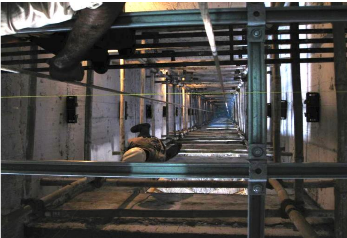
Figure 1 High rise scaffold installation
