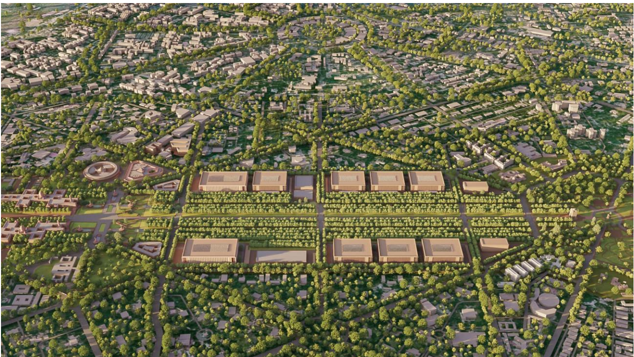
Figure 4 New Central Vista – Aerial view
