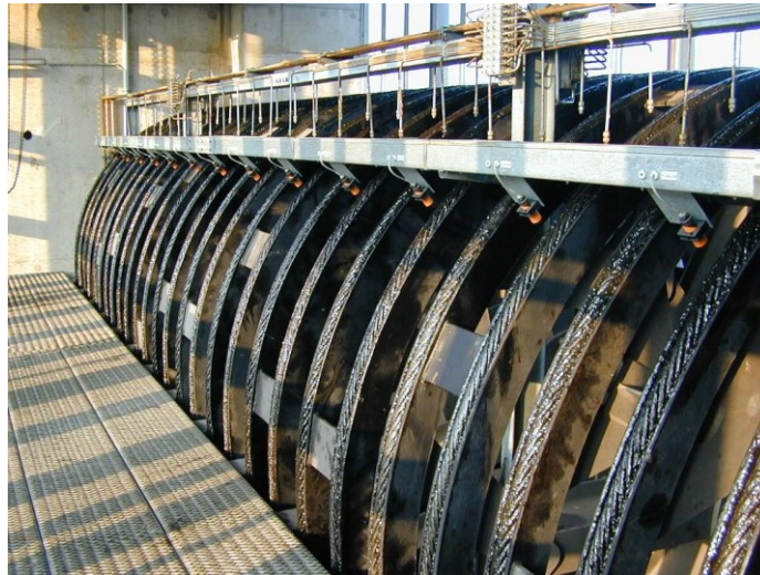
Figure 1 Sheaves of a ship lift
