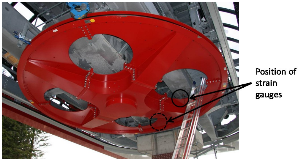
Figure 9 Sheave of a rope way
