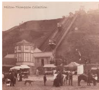
The original inclined lift
