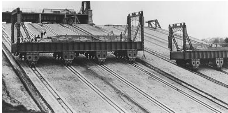
Fig 3: Foxton Inclined Plane under construction
