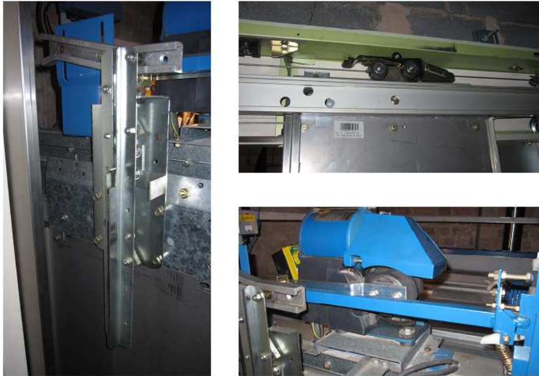
Figure 4: Jobsite survey pictures – source Sematic
