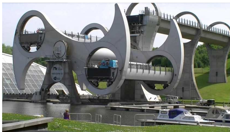
Fig 5: Falkirk Wheel during operation
