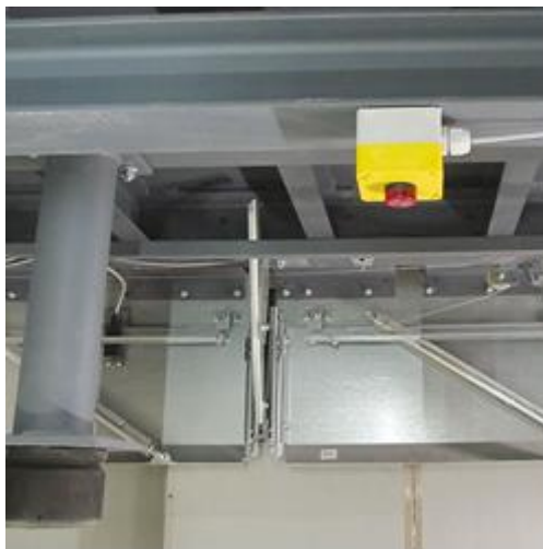
Figure 5: Flashing light with audible alarm
