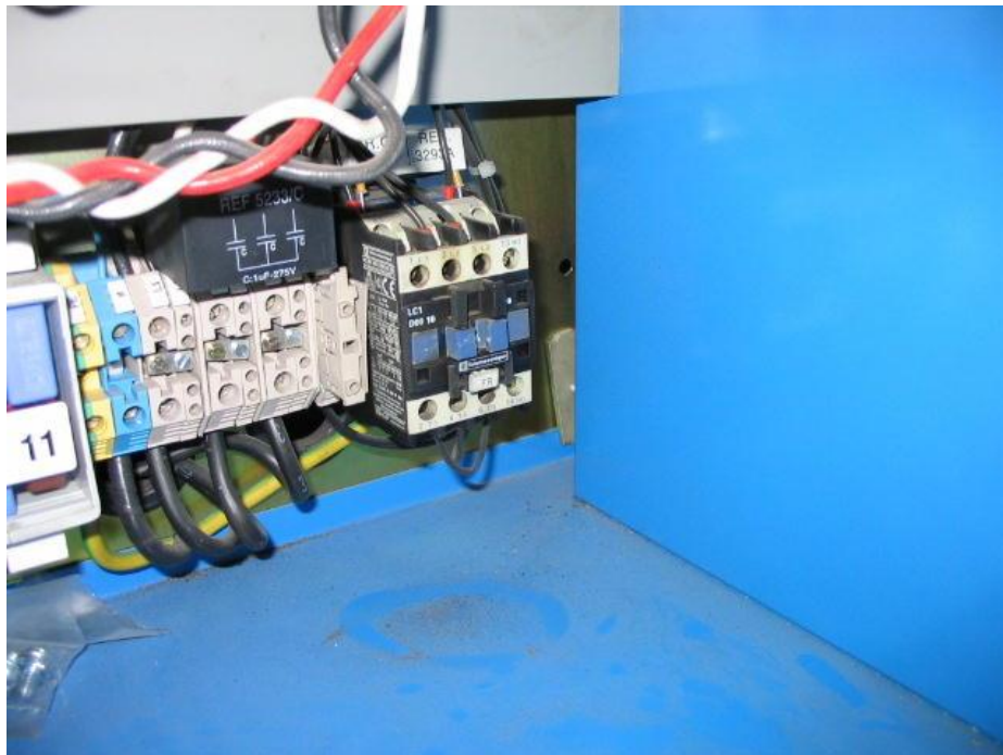
Photograph 2 Build up of carbon dust under the brake contactor indicating oncoming problems.
