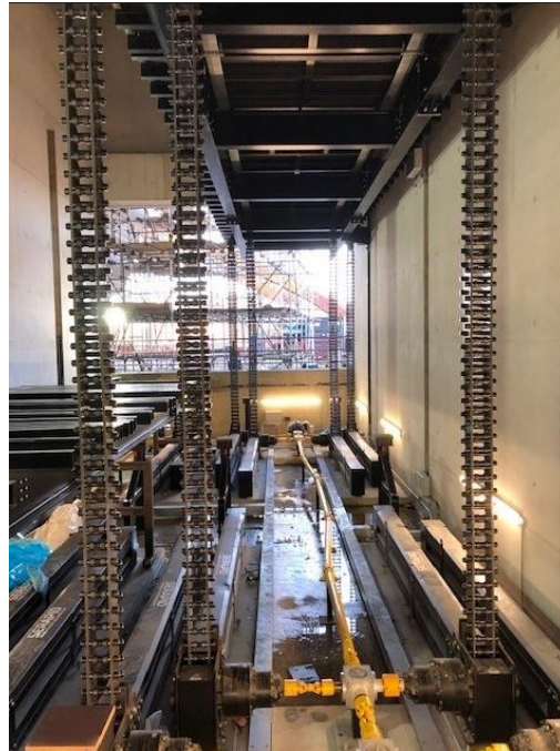
Figure 6 Underneath rigid chain system (during construction)
