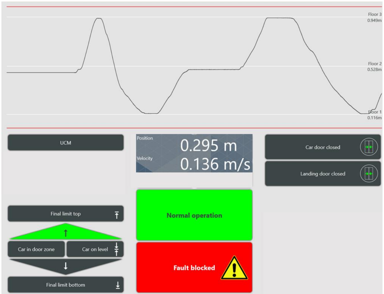
Figure 3 Current lift position, velocity, trip pattern, incl. trip status [travelling upwards] and additional status information of a 3-floor lift
