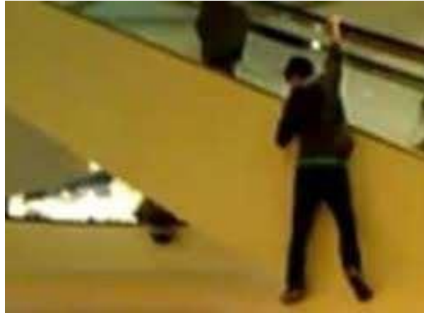
Photo 4: Youth holding onto handrail external to the step band
