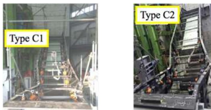
Figure 11 Deformation state of the type C1 and C2 escalator truss
