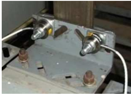
Figure 6: Donut shape load cells installation [2]
