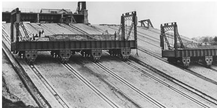
Fig 3: Foxton Inclined Plane under construction
