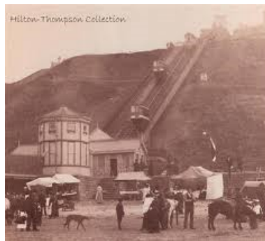
The original inclined lift
