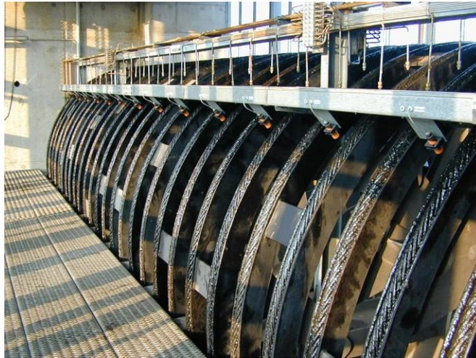
**Figure 1 Sheaves of a ship lift**
