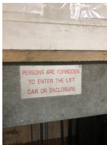
Photograph 1: Typical Sign on a Landing
